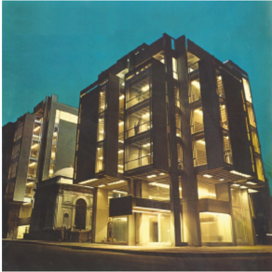
Figure 15. View of the Istanbul Reklam Building [Irexpo introductory booklet, authors archive]
