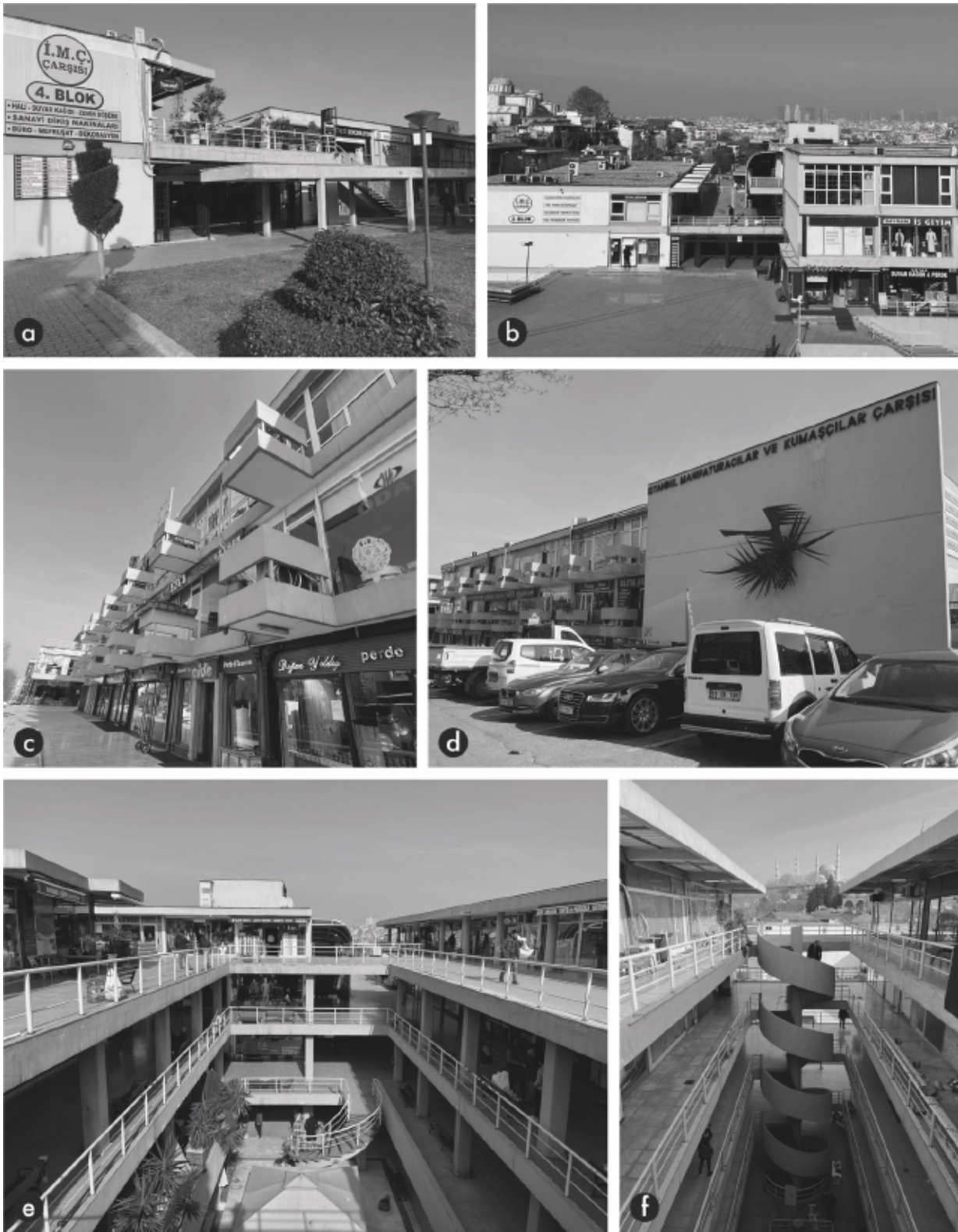
Figure 8. Manifaturaçlar Retail Center; (a) Block 4, (b) Block 2, (c) façade of Block 1, (d) metal relief by Kuzgun Acar, (e) courtyard of Block 1, (f) courtyard of Block 1 (authors archive, 2022)
