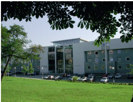
Figure 5. Part of Campus of the Brno Technological University “Pod Palackého vrchem” in Královo Pole quarter
